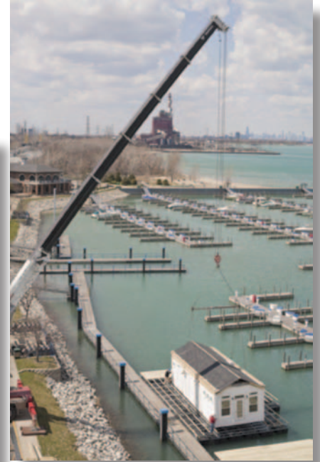
Each of the two bathhouses weighs 39,000 pounds. A crane was used to place the structures onto the floats designed and built by Merco Marine.
